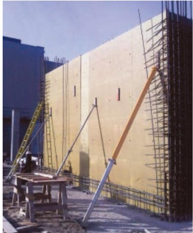
*Hi-Flow Concrete Forms - balanced Douglas fir construction resulting in a strong and stable panel.*
