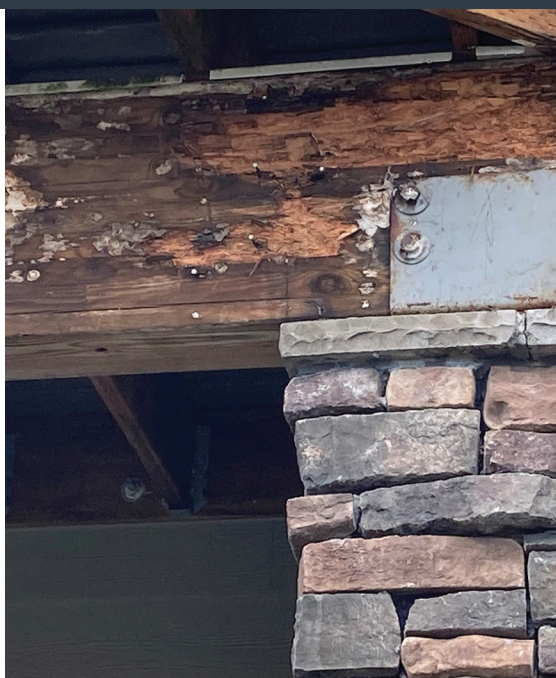
Example of a treated beam that was wrapped. Moisture was trapped and accelerated deterioration.
